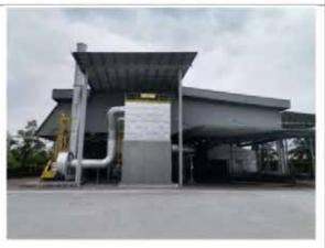
Dust collector serves to protect to remove debris and gas removal as component process in a recycling of scrap waste.
