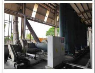
A scrubber water treatment unit functions to remove polycyclic aromatic hydrocarbons (PAH), particulate matter (PM), and other unwanted particles. This process benefits the environment by fighting ocean acidification
