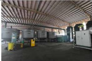
Neutralization tanks are used to alter the pH level of corrosive waste drainage—by dilution or chemical neutralization—so the treated effluent can be safely discharged into sanitary sewer systems in compliance with local regulations.
